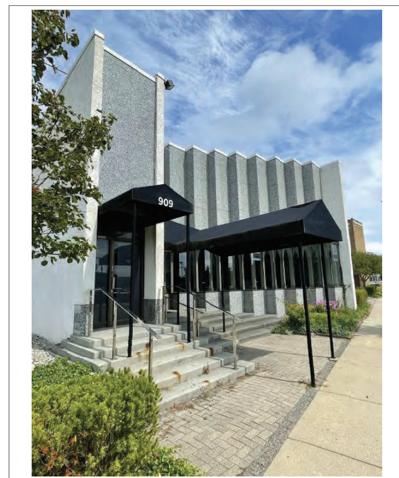
3 HAYNES ST. (SOUTH SIDE) LOOKING EAST - EXISTING TO BE REMOVED
